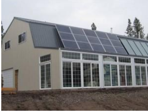
Rooftop solar panels
